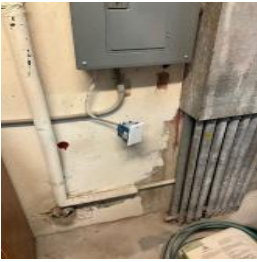
Maintenance room ground floor
