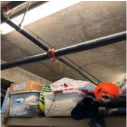
Apartment 401 residential storage locker
