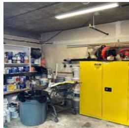
Paint room ground level
