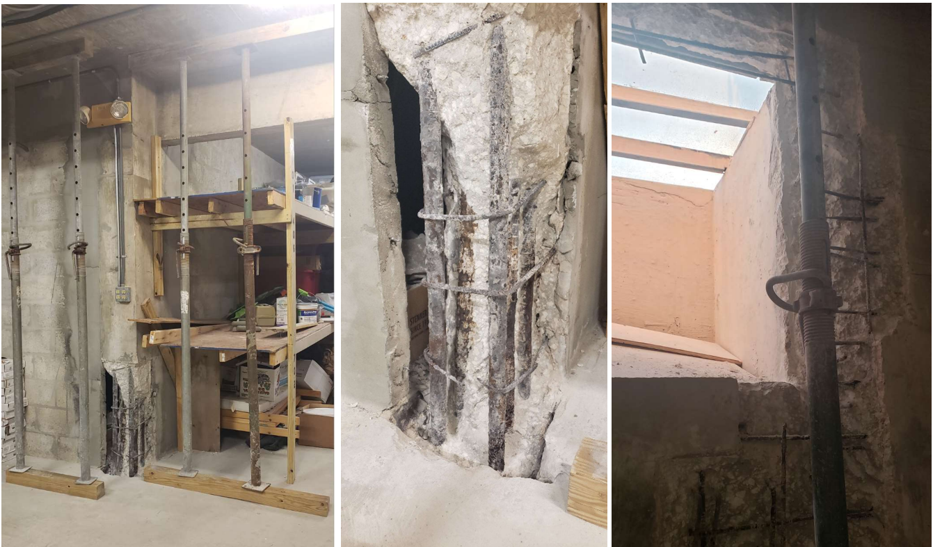
Storage area shoring installed for column repair. Rusted Rebar and stirrups in column. Storage window removed and wall repairs in progress.
