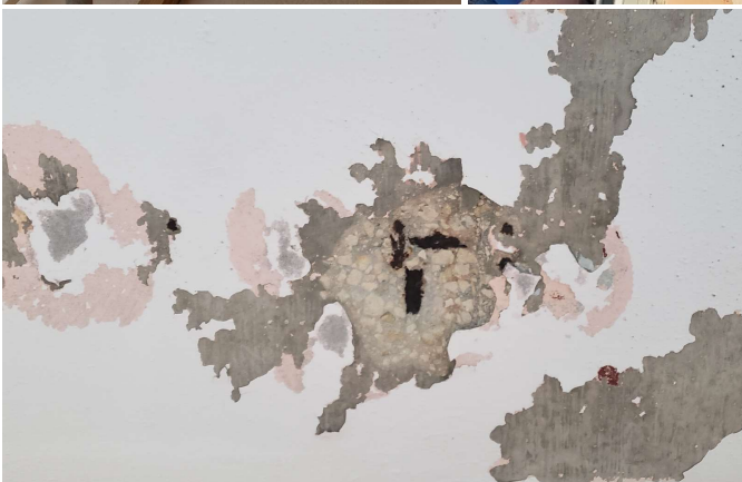
After pressure washing – exposed areas of rusted rebar, rebar supports and failing expansion joint.
