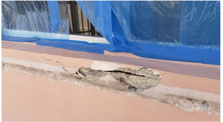
Unit 705 Window – crack identified and rust and corrosion revealed after shutter was removed.
