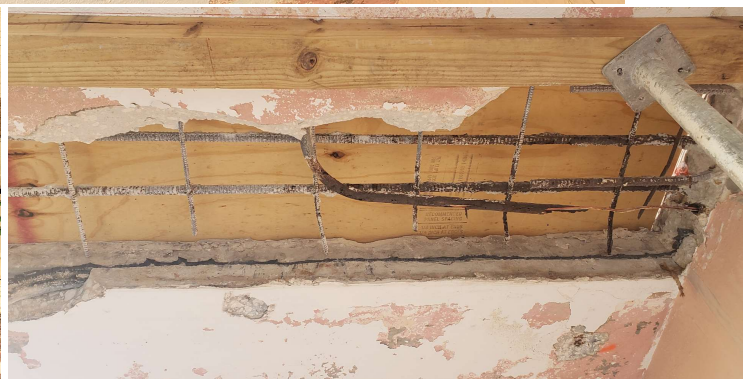
Rusted/corroded conduit and exposed wires in multiple locations. Conduit to be replaced in these areas.
