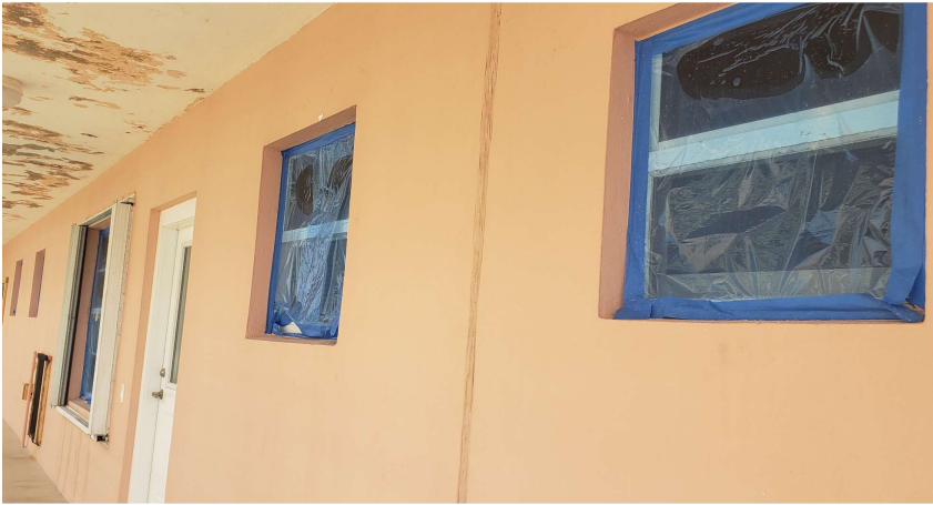
Temporary protection installed on all windows. AC units protected by thick poly.
