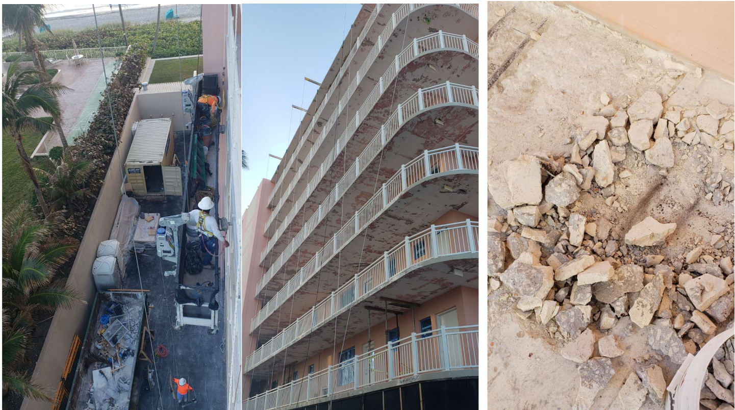
Workers accessing floors via swing stage. Overall view of progress after 2 weeks. Closeup of topping/overlay.
