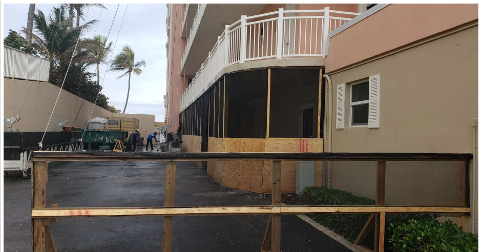
Temporary protection installed at side door for pedestrian access to maintenance, trash, and storage areas.
