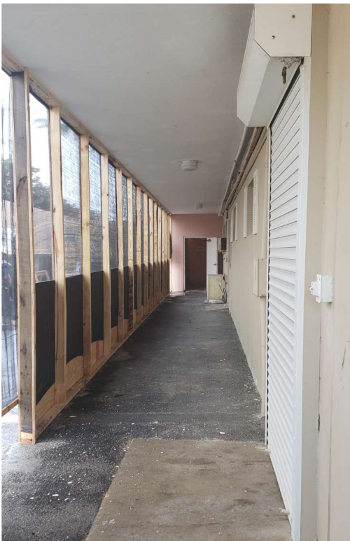
Temporary protection installed at side door for pedestrian access to maintenance, trash, and storage areas.
