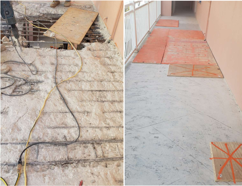
Full depth repair required on 2 nd Floor. Contractor covers exposed/open slab areas with plywood at the end of each day.
