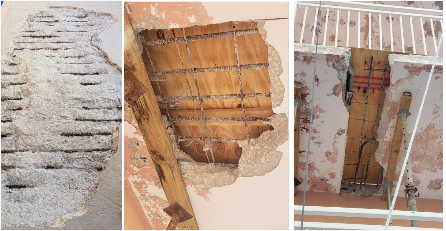
Areas on the 2 nd Floor where concrete rebar is rusted. Full depth repairs will be required in these locations. Note topping slab can be seen in first photo along chipped edge. Very little concrete cover over rusted rebar.
