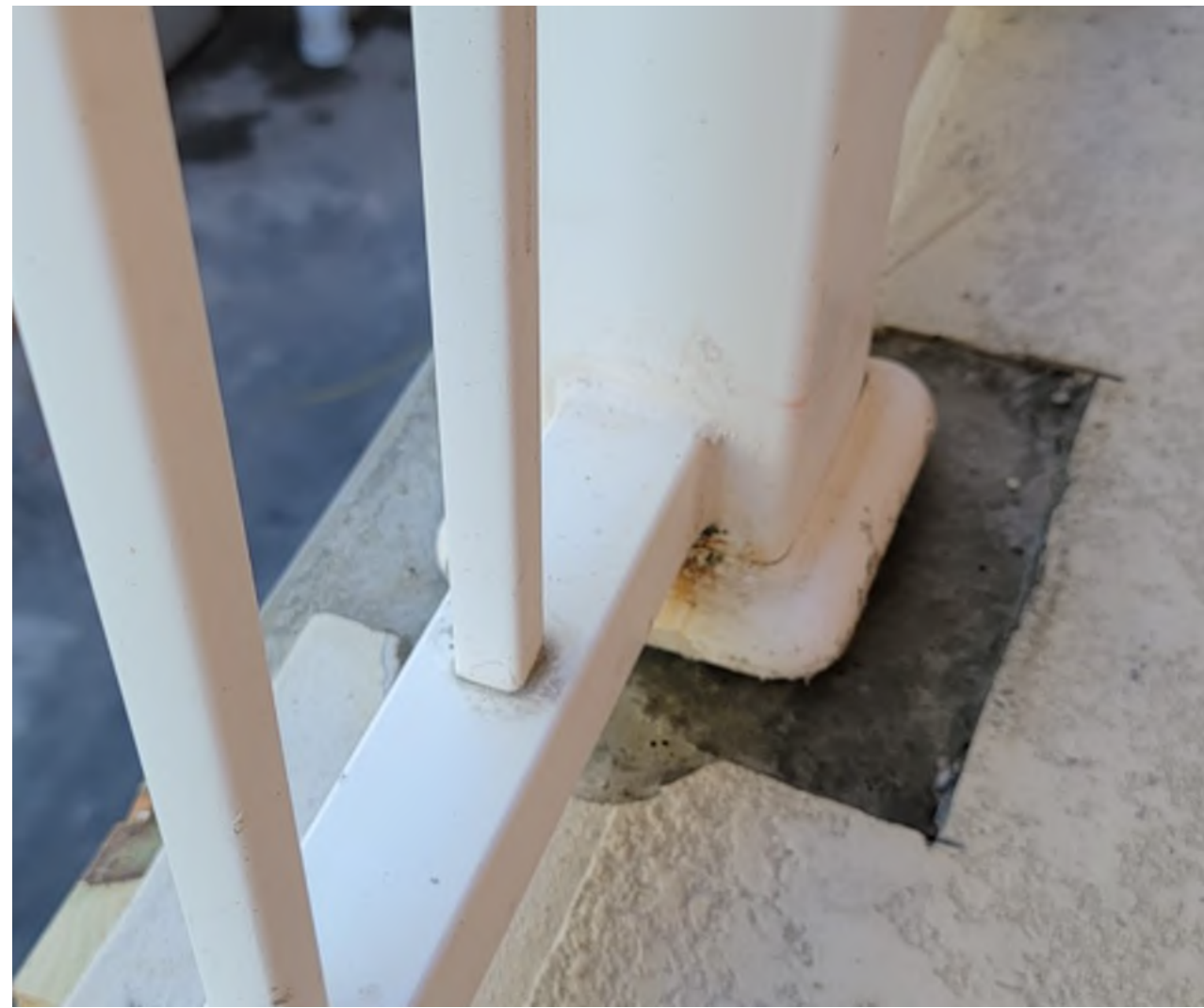
Repair of Rusted Anchors on North Catwalk at Existing Railing
