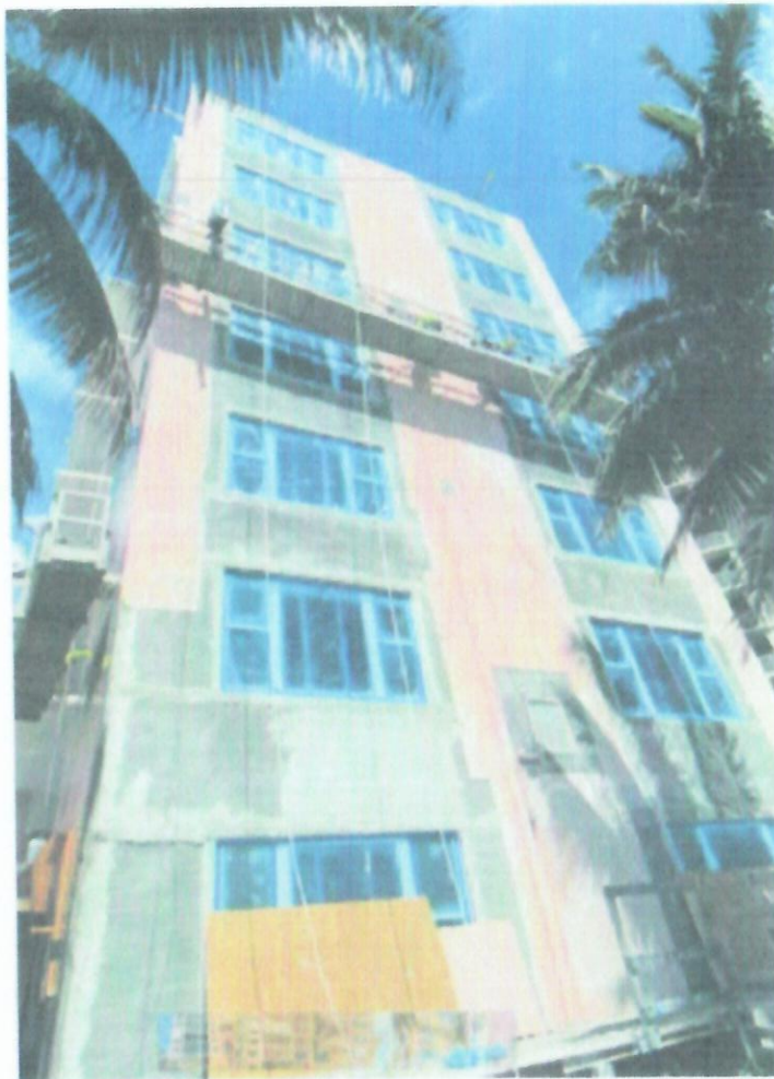
7 STACK East - Windows installed, stucco work ongoing
