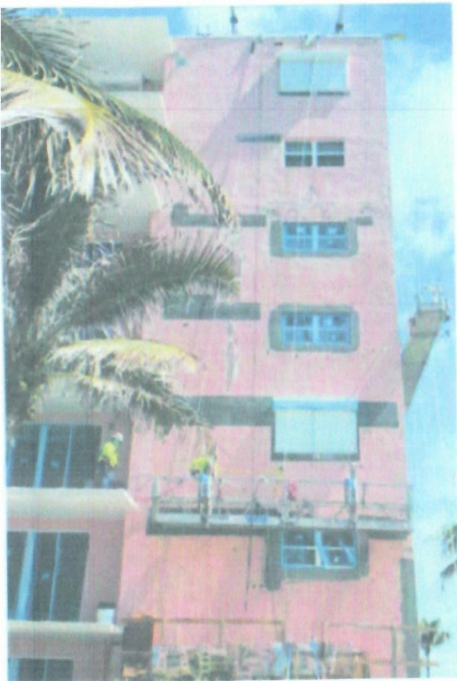
7 STACK South - Windows installed, final painting
