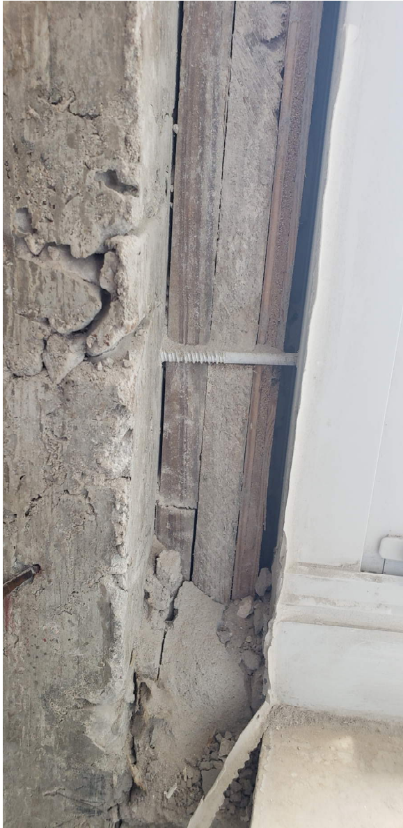
East 7 Stack - Drywall/plaster removal exposing window anchors with little or no embedment into structure at jambs
