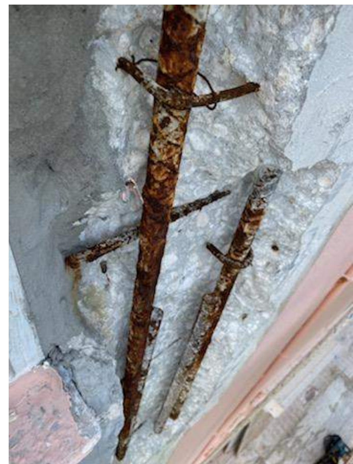
East 7 Stack Wall - Rusted rebar found in columns at windows
