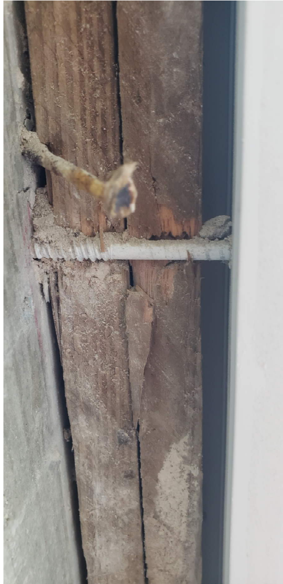
East 7 Stack - Drywall/plaster removal exposing window anchors with little or no embedment into structure at jambs
