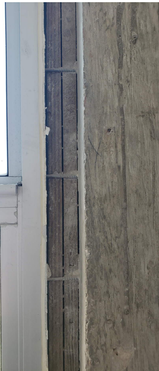
East 7 Stack - Drywall/plaster removal exposing window anchors with little or no embedment into structure at jambs
