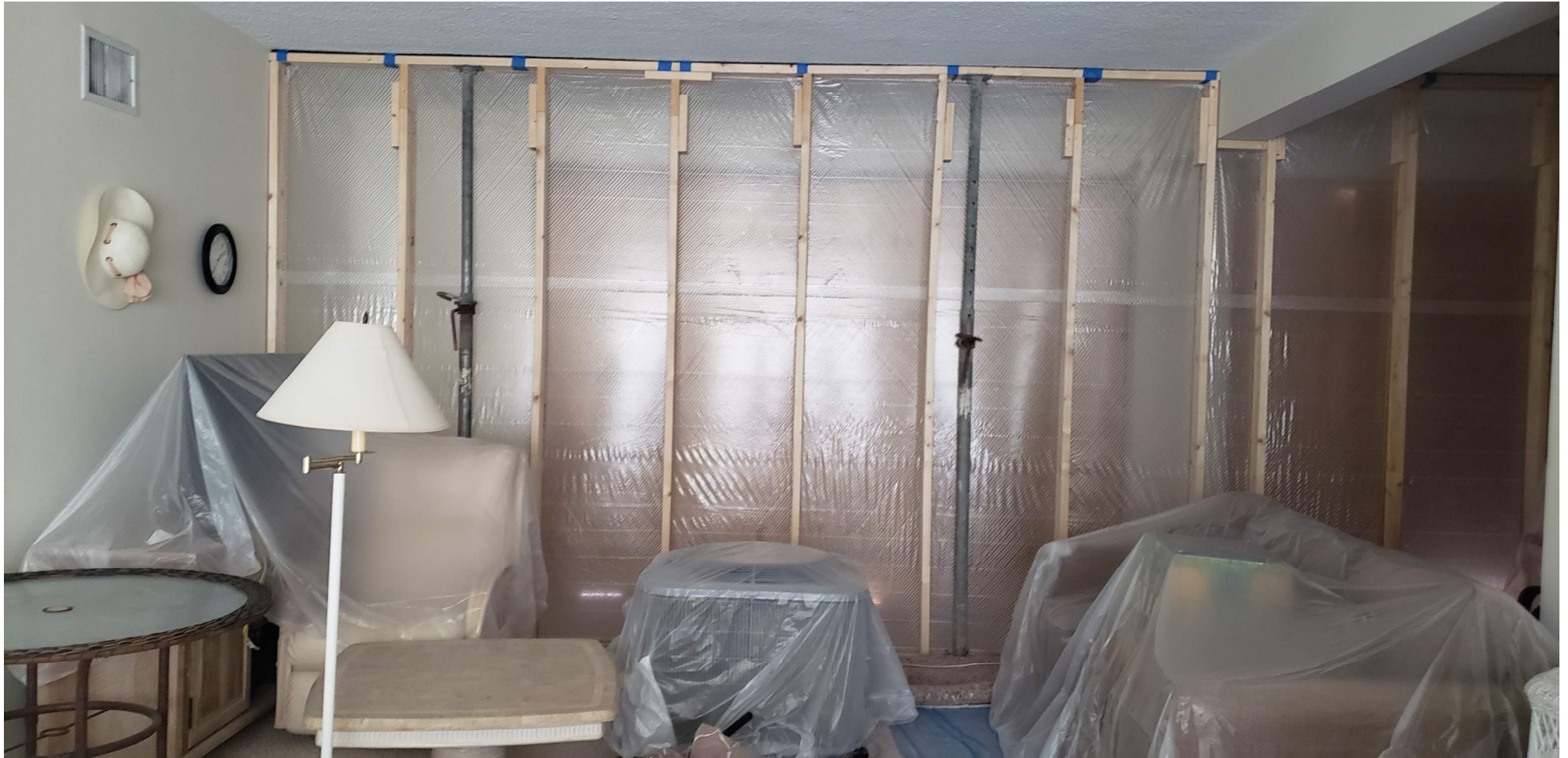
7 Stack - Interior dust walls built inside apartments at sliding glass doors
