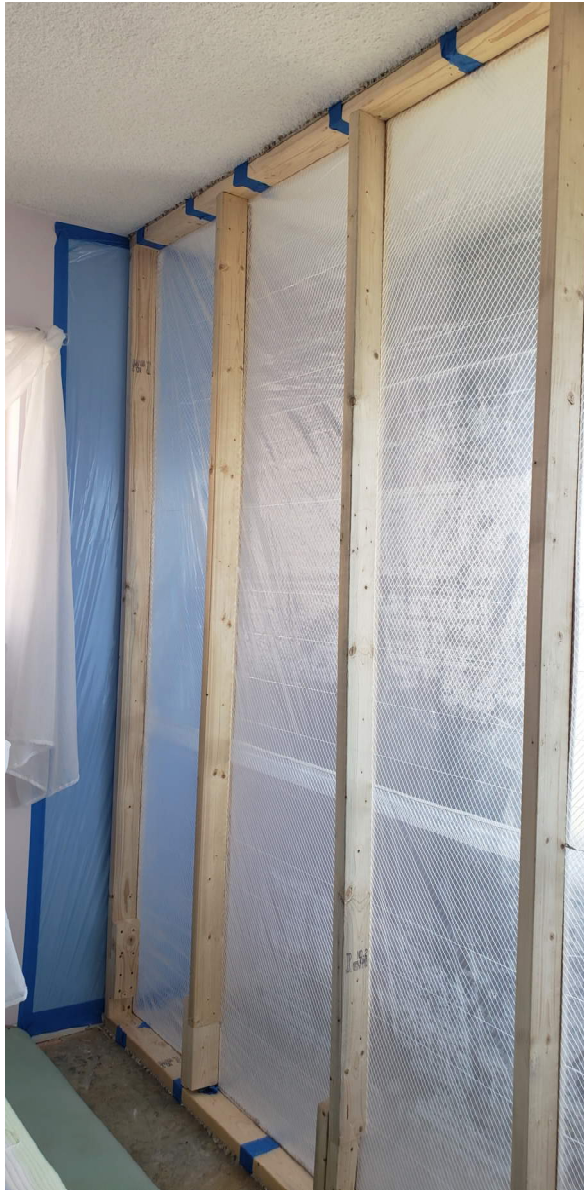
East 7 Stack - Interior dust walls built inside apartments at windows
