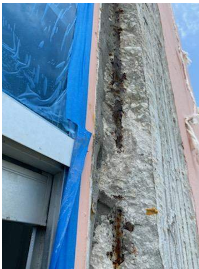
East 7 Stack Wall - Rusted rebar found in columns at windows
