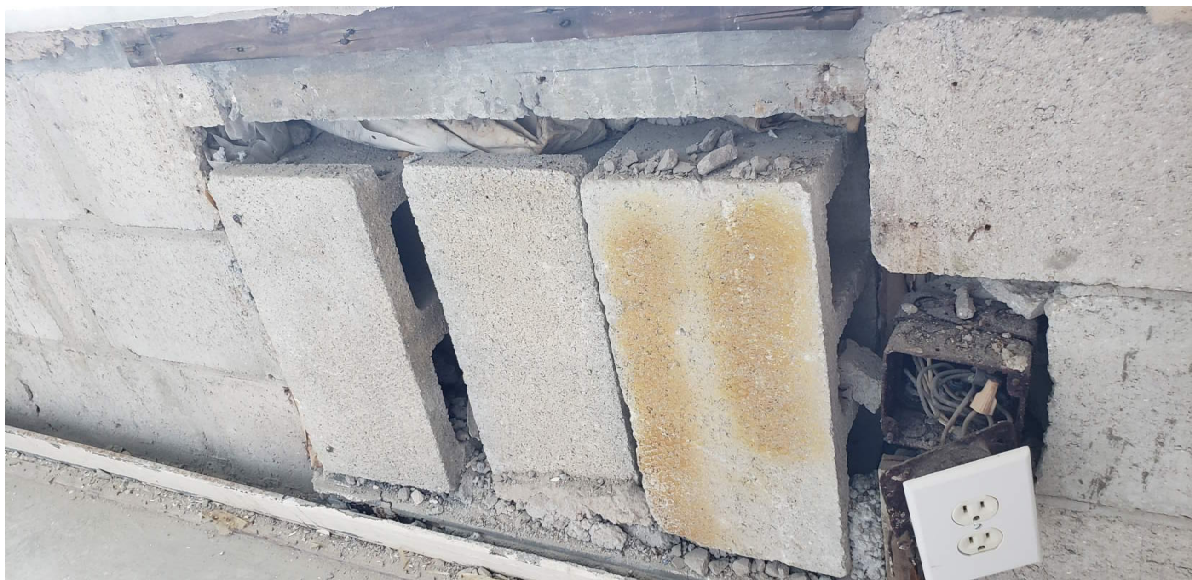
East 7 Stack - CMU fill-in at window ACs
