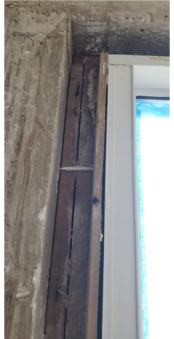
East 7 Stack - Drywall/plaster removal exposing window anchors with little or no embedment into structure at jambs
