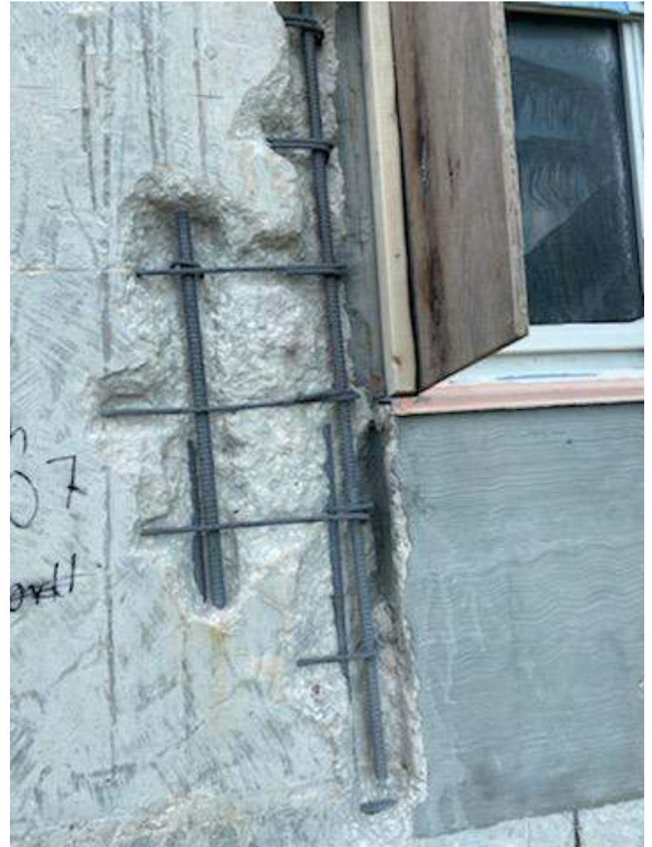
East 7 Stack Wall - Rusted rebar repaired in columns at windows
