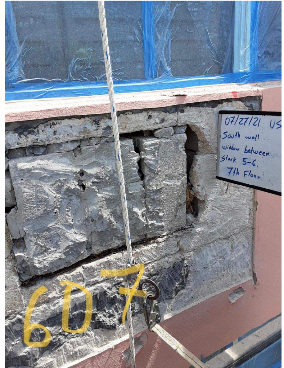
East 7 Stack - Old Window AC fill-in beneath windows
