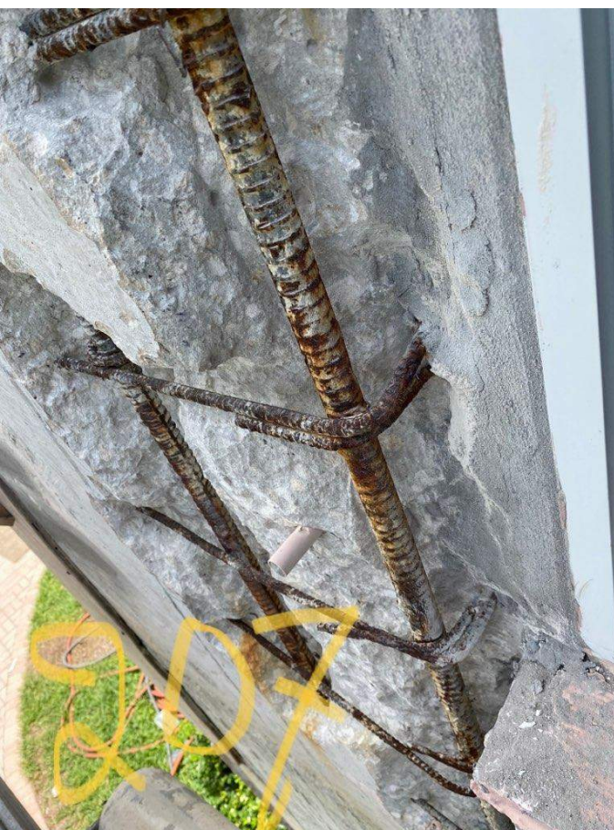
East 7 Stack Wall - Rusted rebar found in columns at windows
