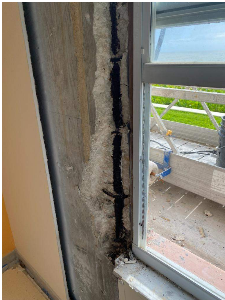
East 7 Stack - Drywall/plaster removal exposing rusted rebar in columns at interior windows
