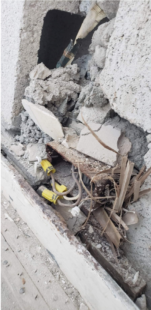
East 7 Stack - Rusted electrical boxes, conduit and wiring under windows
