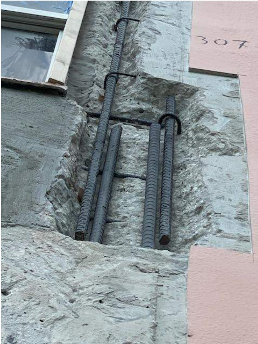
East 7 Stack Wall - Rusted rebar repaired in columns at windows
