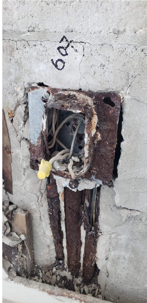
East 7 Stack - Rusted electrical boxes, conduit and wiring under windows
