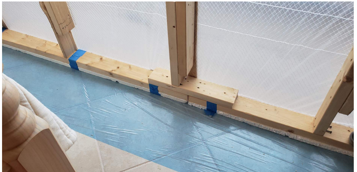
East 7 Stack - Interior dust walls built inside apartments at windows
