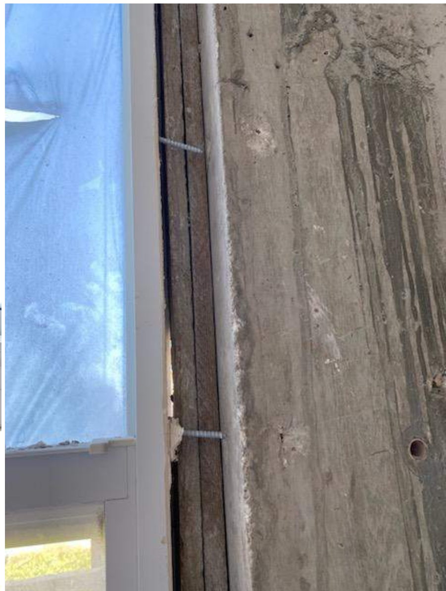
East 7 Stack - Drywall/plaster removal exposing window anchors with little or no embedment into structure at jambs
