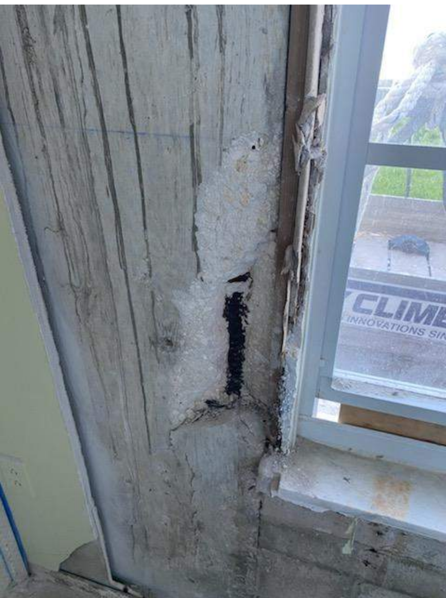
East 7 Stack - Drywall/plaster removal exposing rusted rebar in columns at interior windows
