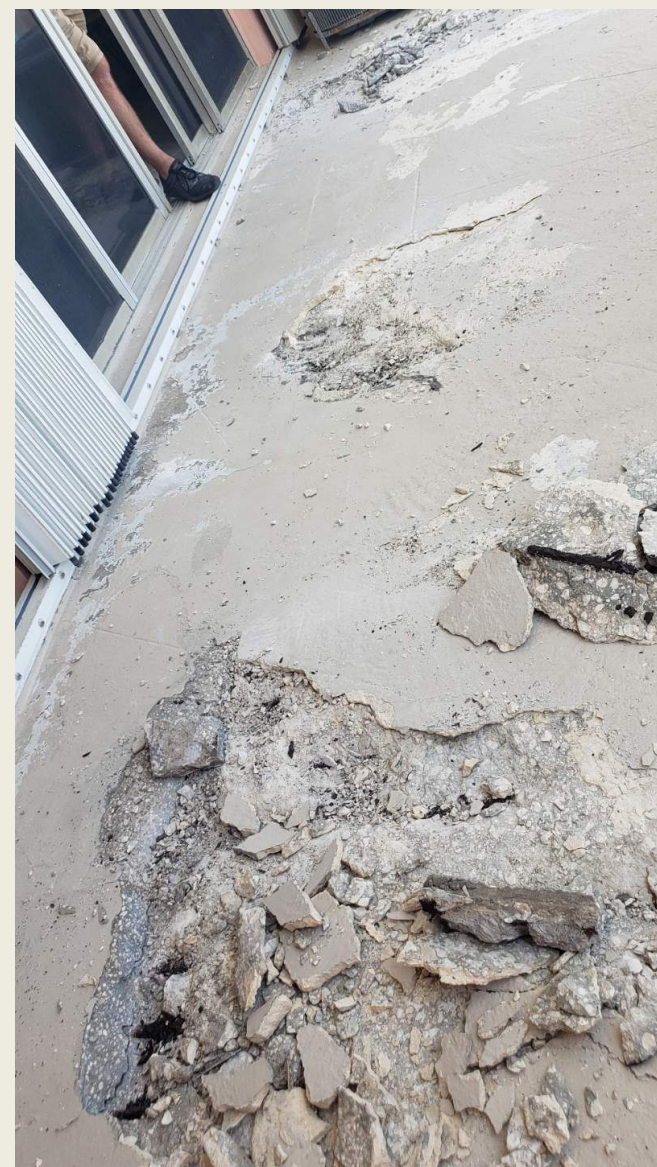
Balcony Corrosion
