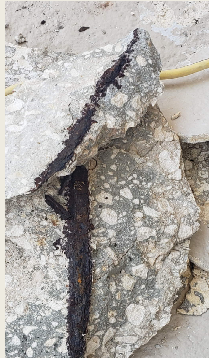
Balcony Corrosion
