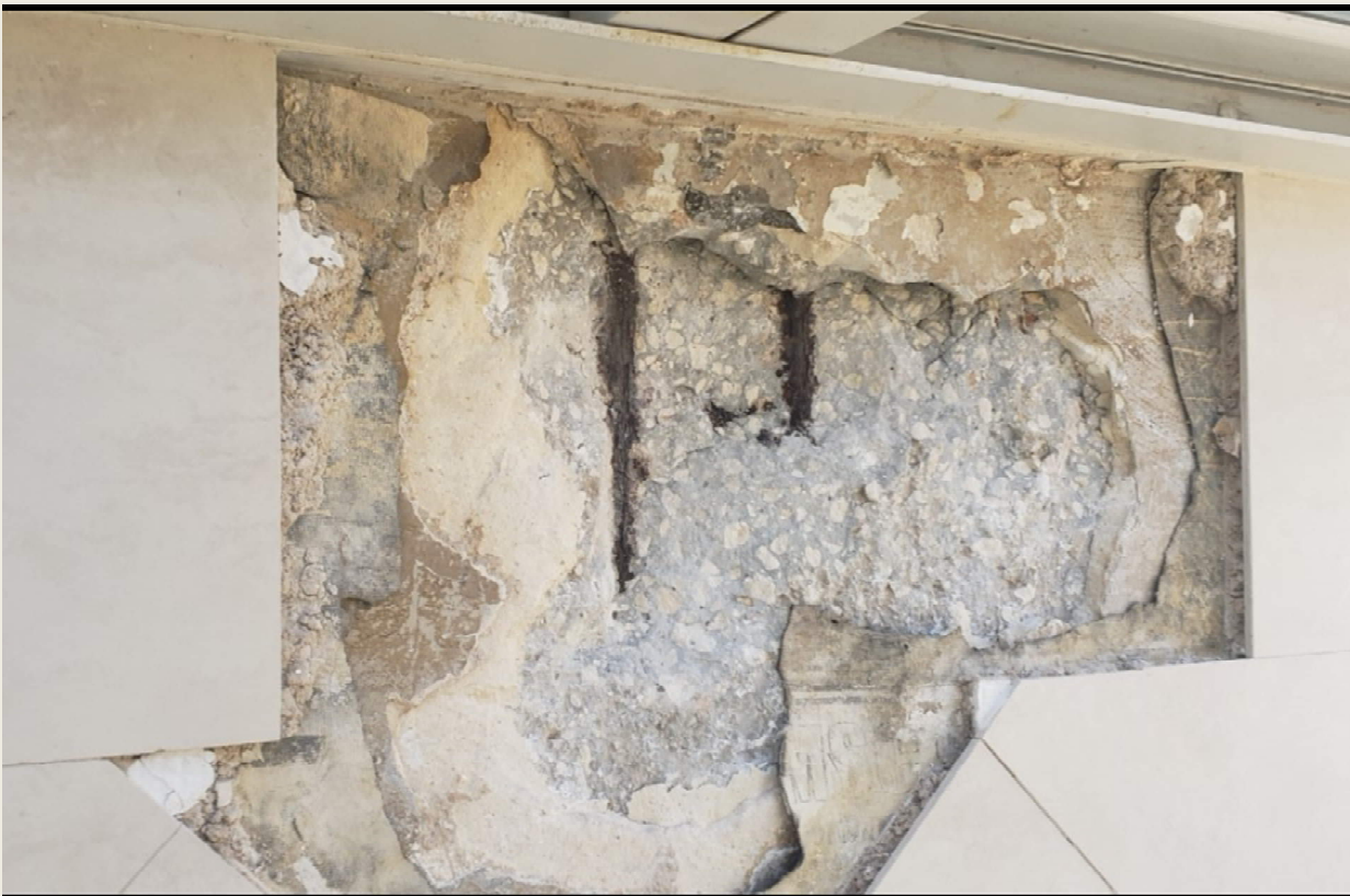
Balcony Corrosion At Sliding Glass Door
