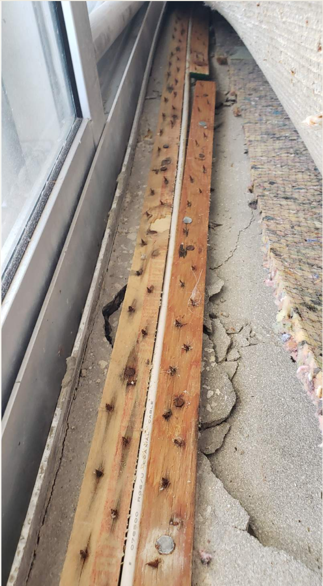
Balcony Corrosion
