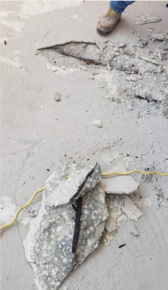
Balcony Corrosion
