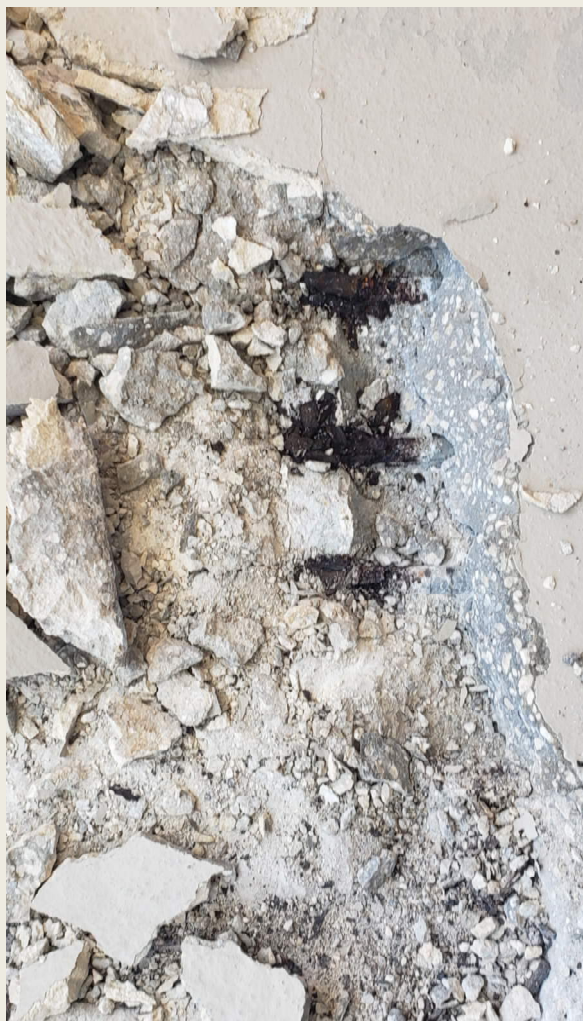
Balcony Corrosion
