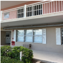
Fire pump water supply piping
