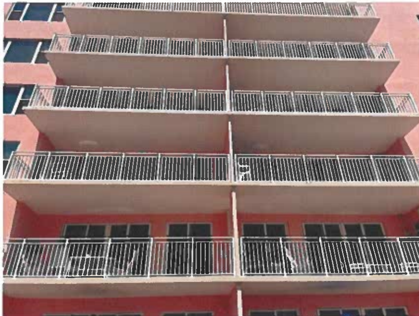
balcony stacks 06/07 floors, walls, ceilings, and edges without cracks and spalls
