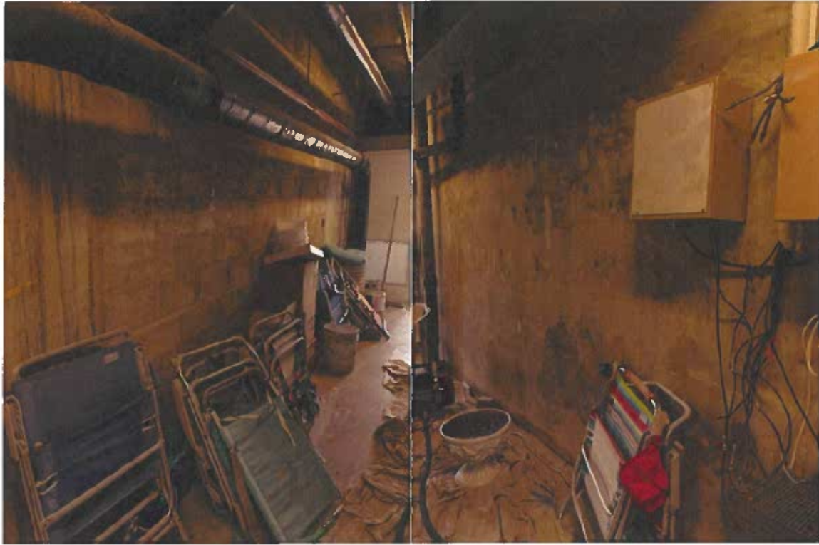
s.w.storage room – south floor, wall, ceiling, and floor without cracks s.w. storage room – north shear wall, floor & ceiling without cracks
