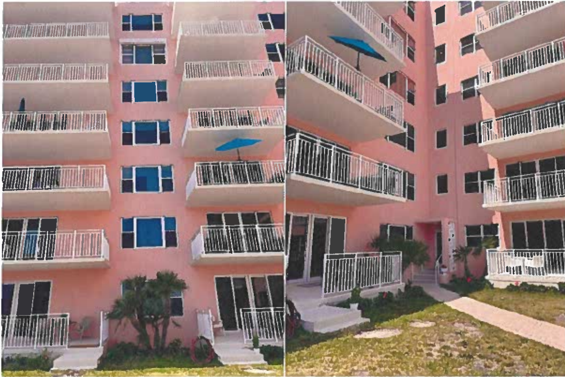
Balcony stack 02/03 floors, ceiling, edges & walls without cracks & spalls Balcony 04/05 floors, ceiling, edges & walls without cracks & spalls
