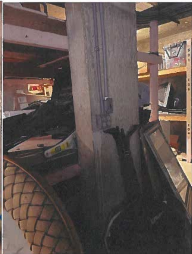
n.e. storage room – column and ceiling without cracks
