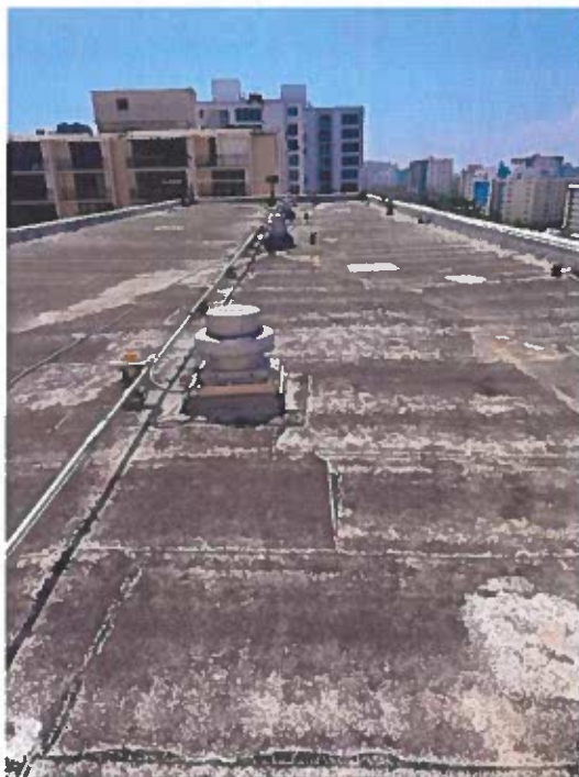
west wing – built-up roofing membrane
