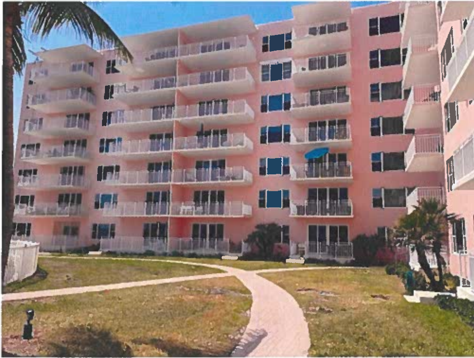
east elevation – all balconies at stacks 01 – 04 finished without balcony enclosures
