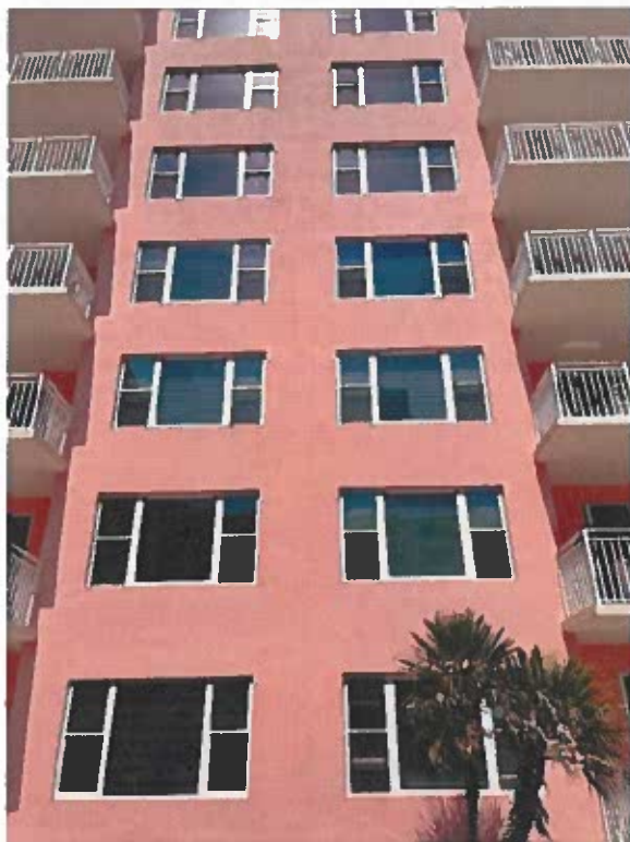
south elevation – stack 05/06 wall without cracks & spalls
