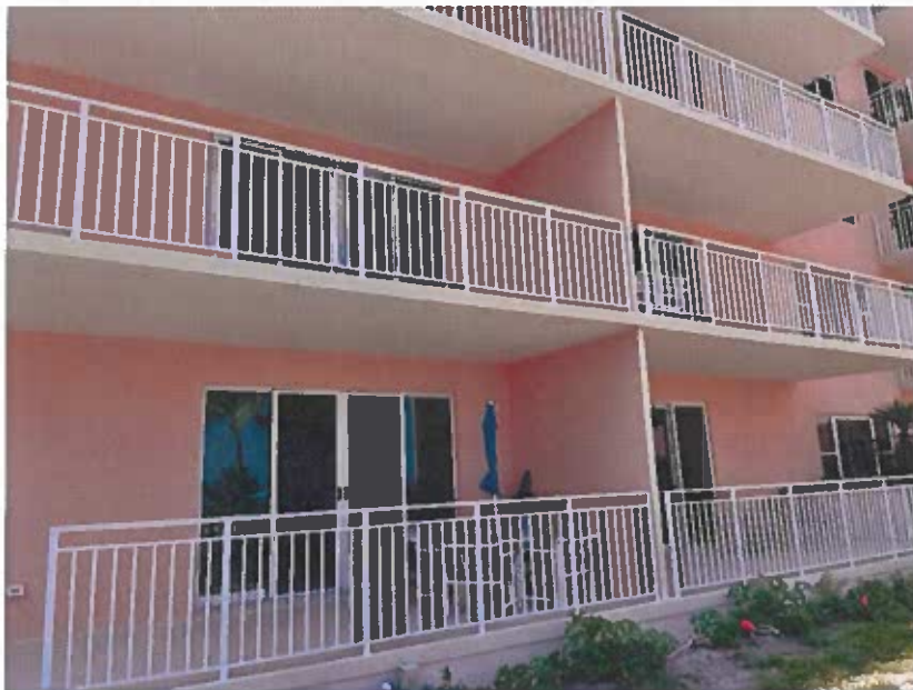
east elevation – 02/03 balcony floors, ceilings, and edges without cracks and spalls
