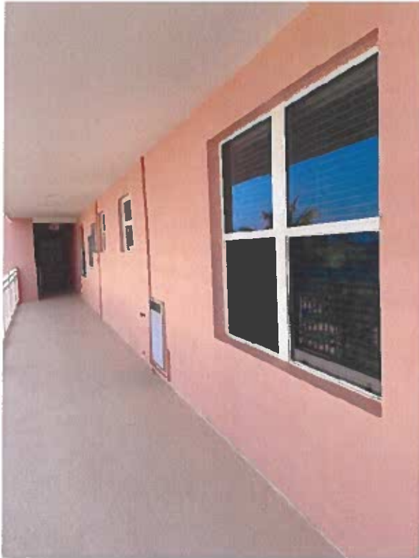
4th floor catwalk floor & ceiling without cracks and spalls
