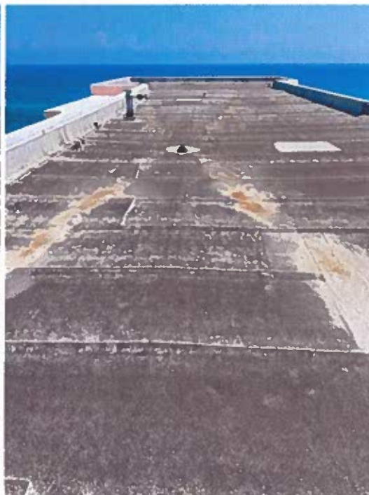
north wing – built-up roofing membrane
