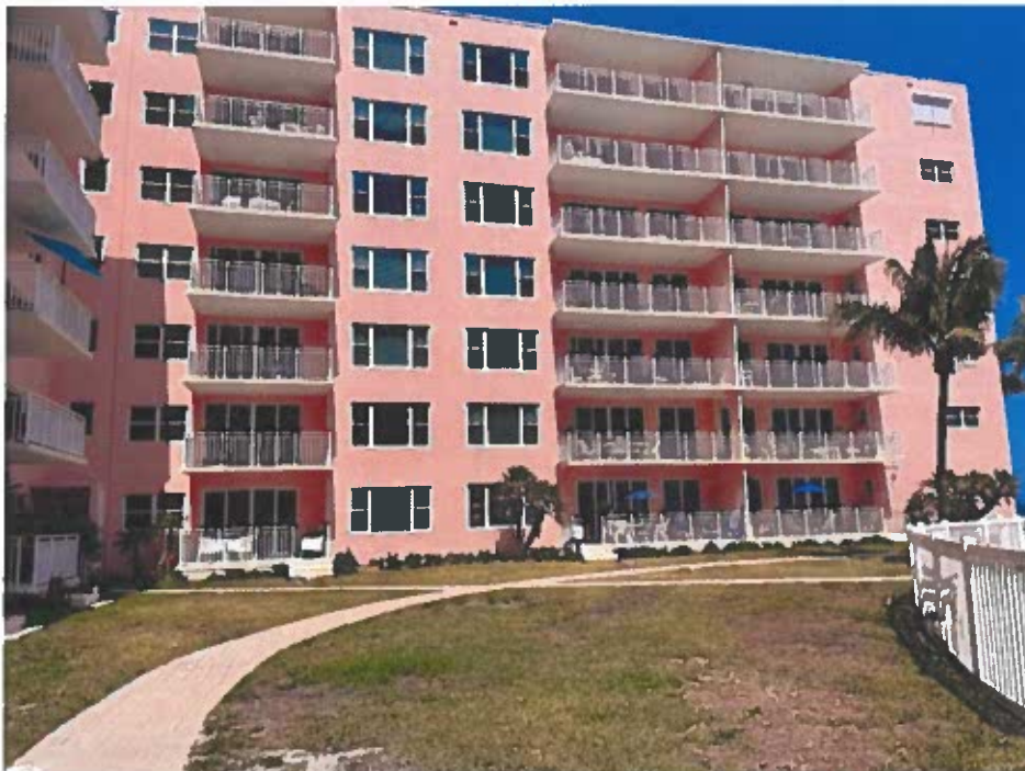
south elevation – all balconies at stacks 05 – 07 finished without balcony enclosures
