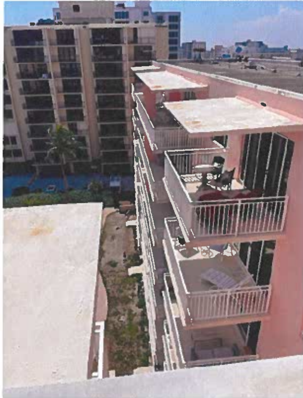
balcony stack 04, 03/02,01 floors, walls, ceiling without cracks & spalls
