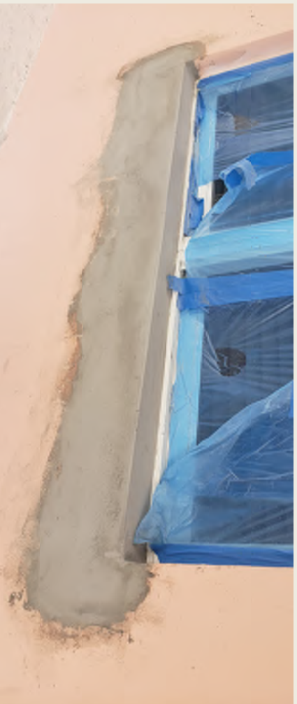
Stucco on Repaired Sills, Thresholds and Columns
