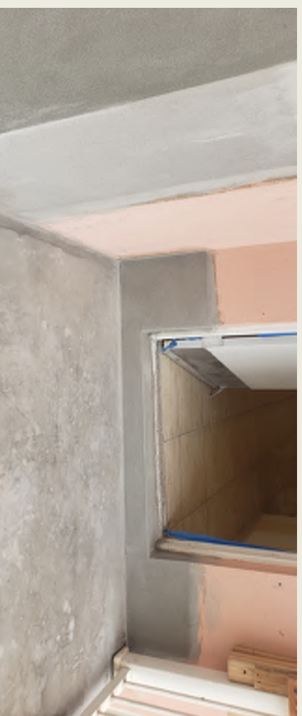
Stucco on Repaired Sills, Thresholds and Columns
